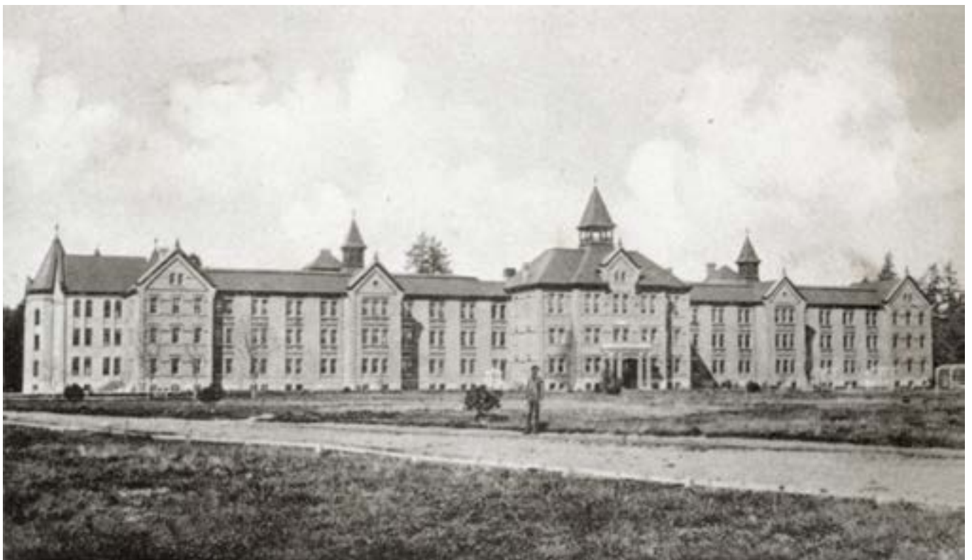
Western State Hospital, Pierce, Washington
